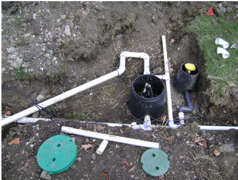
Landscape Irrigation System Construction
