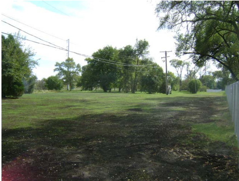
Staging Area Restoration
