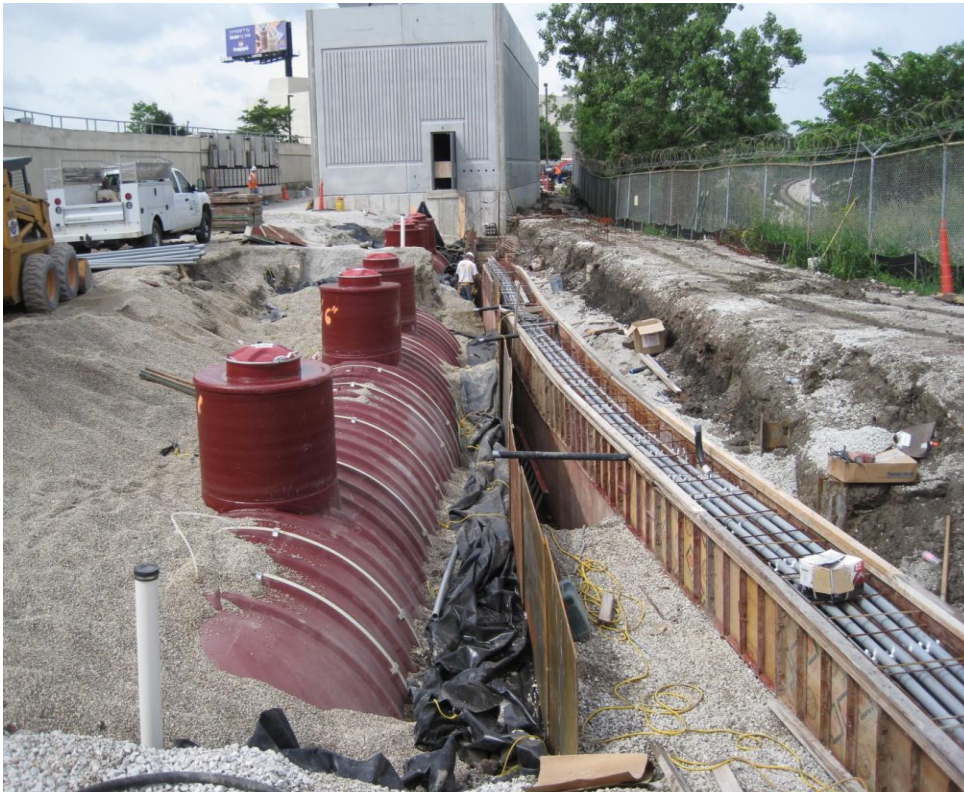
Duct Bank Between Electrical and Generator Building
