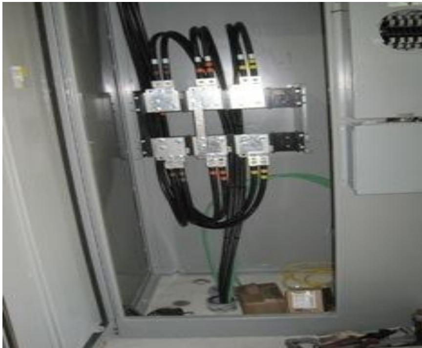
Cable Termination in CT Meter Cabinet
