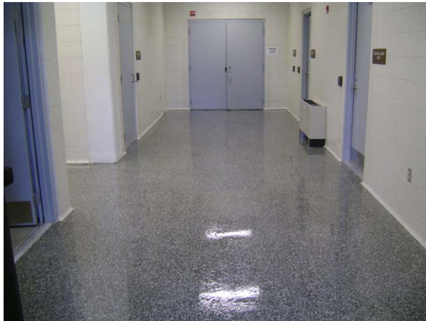
Lobby Floor Progress
