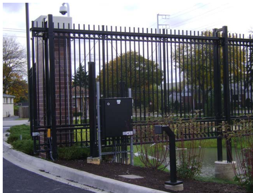
Security Camera, Infrared Security Tower & Gate Operator
