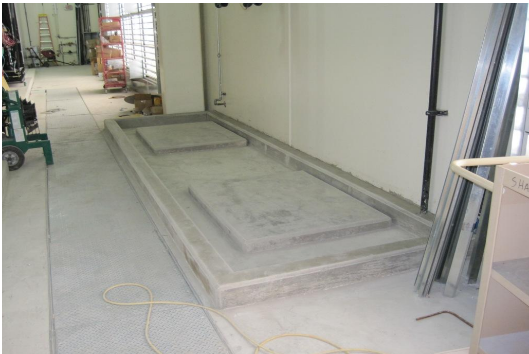
Day Tank Equipment Pads and Curb in Generator Building
