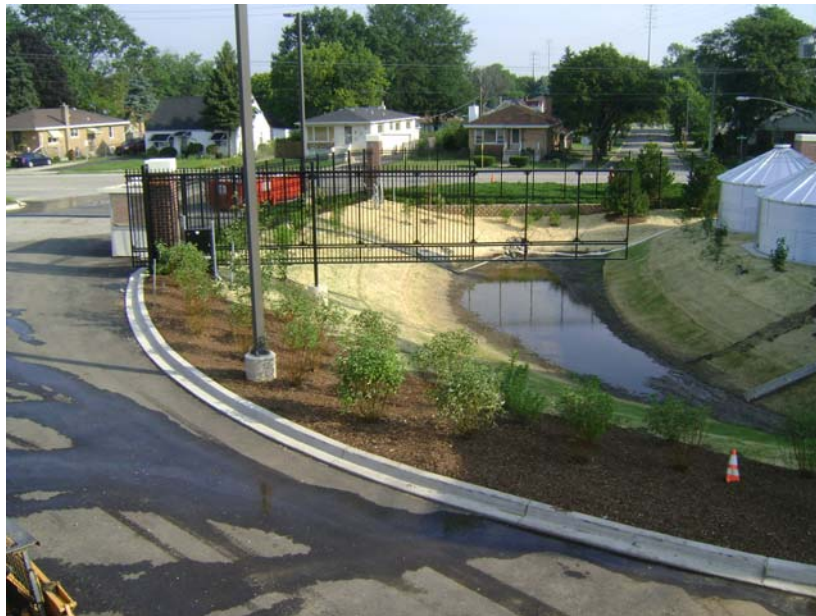
Retention Basin Progress
