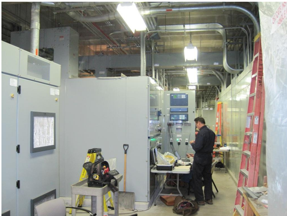
Modification to Existing Switchgear
