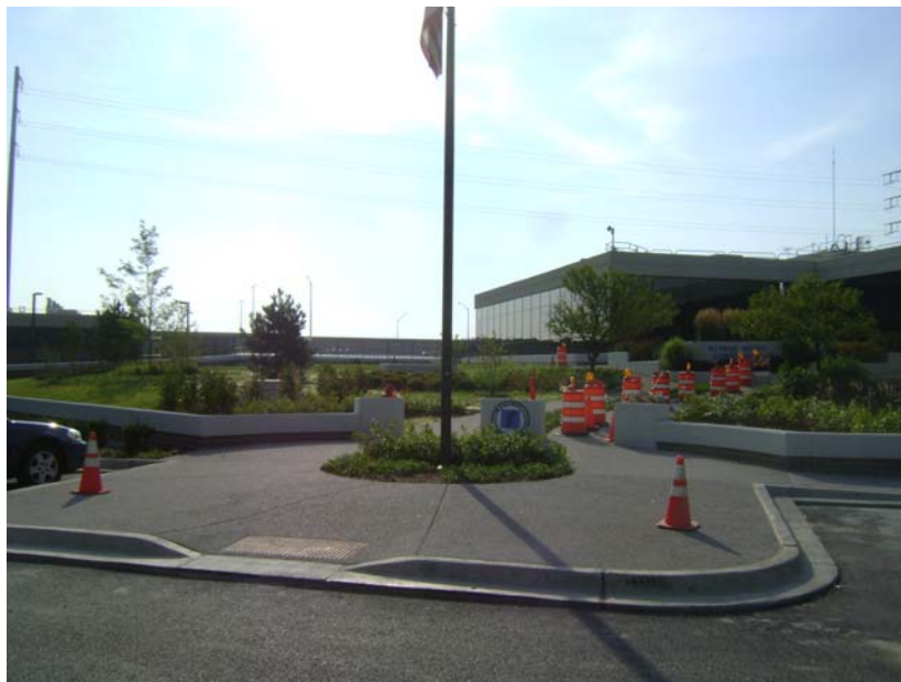
Front Entrance Progress
