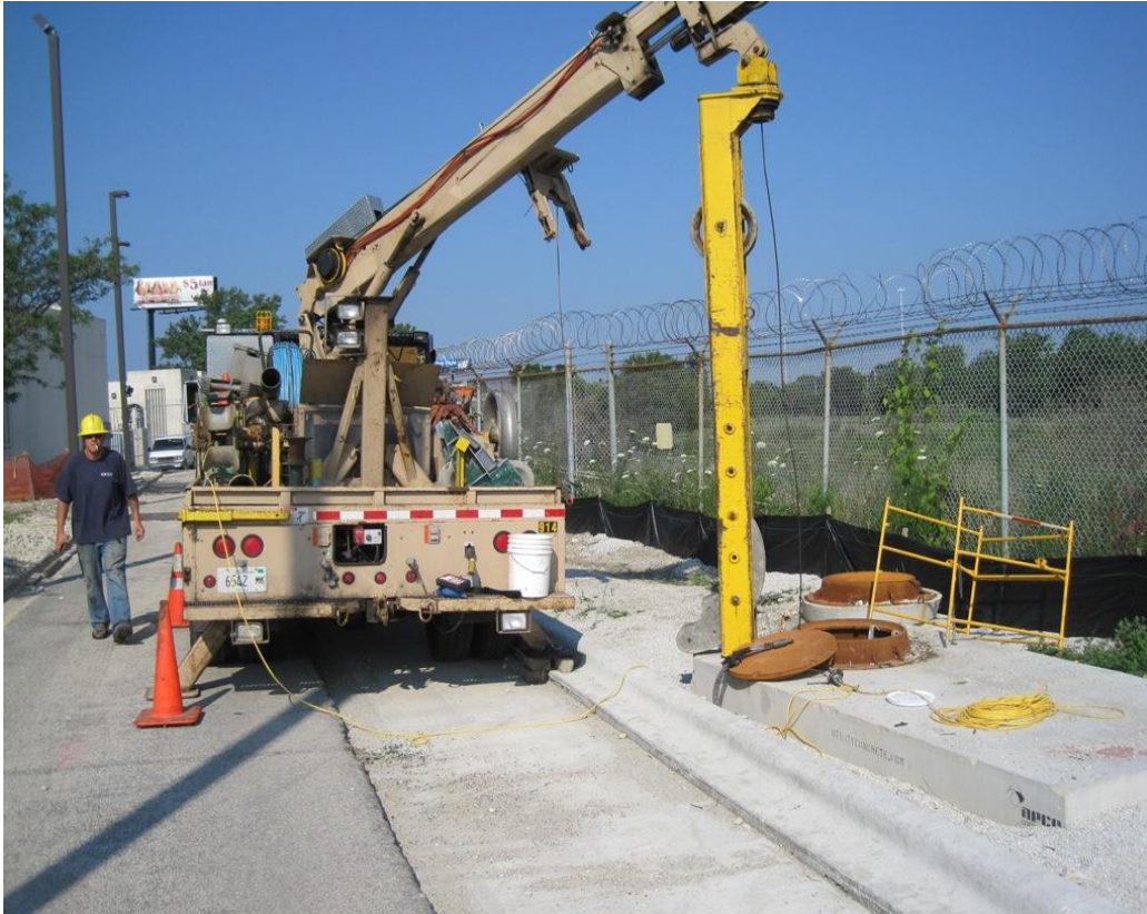
Day Tank Equipment Pads and Curb in Generator Building
