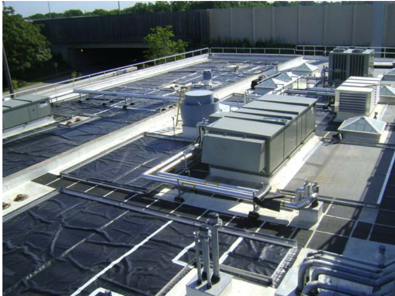
Vegetative Green Roof Progress
