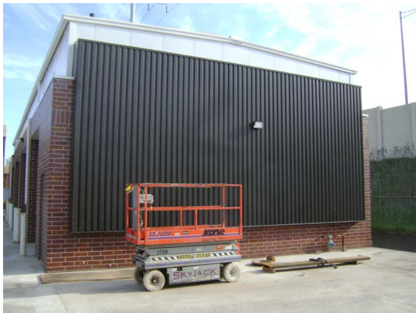
Solar Wall Installation
