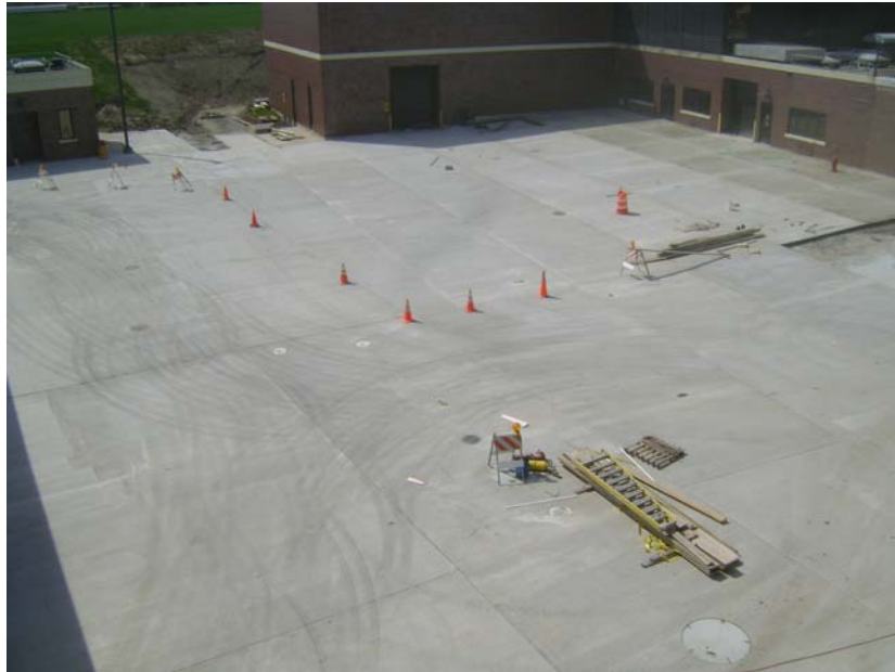
Parking Lot Progress
