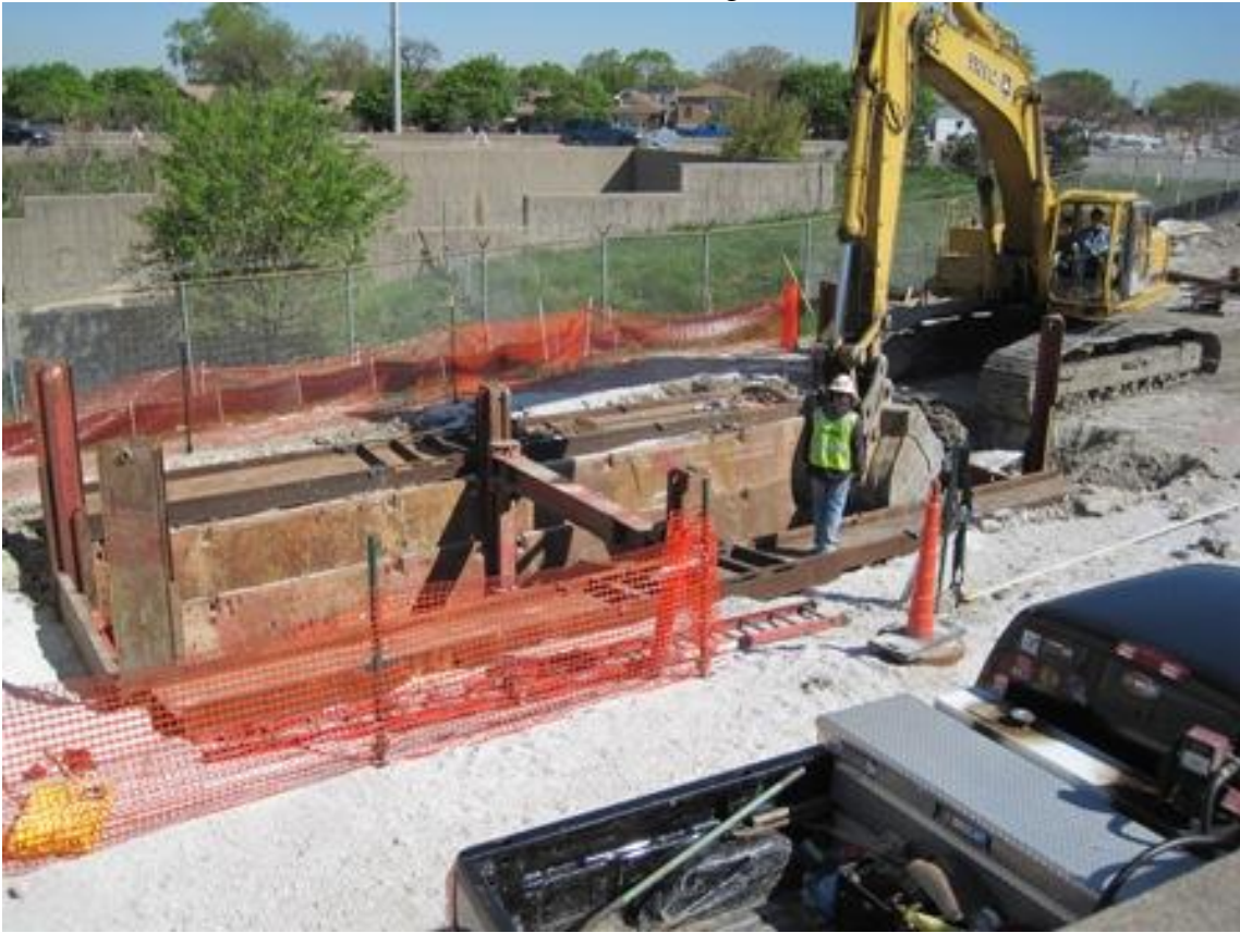
Start of excavation for 10,000 gallon fuel tank
