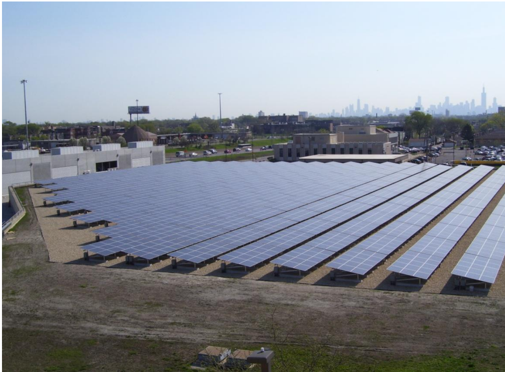
Final leveled off PV Panels
