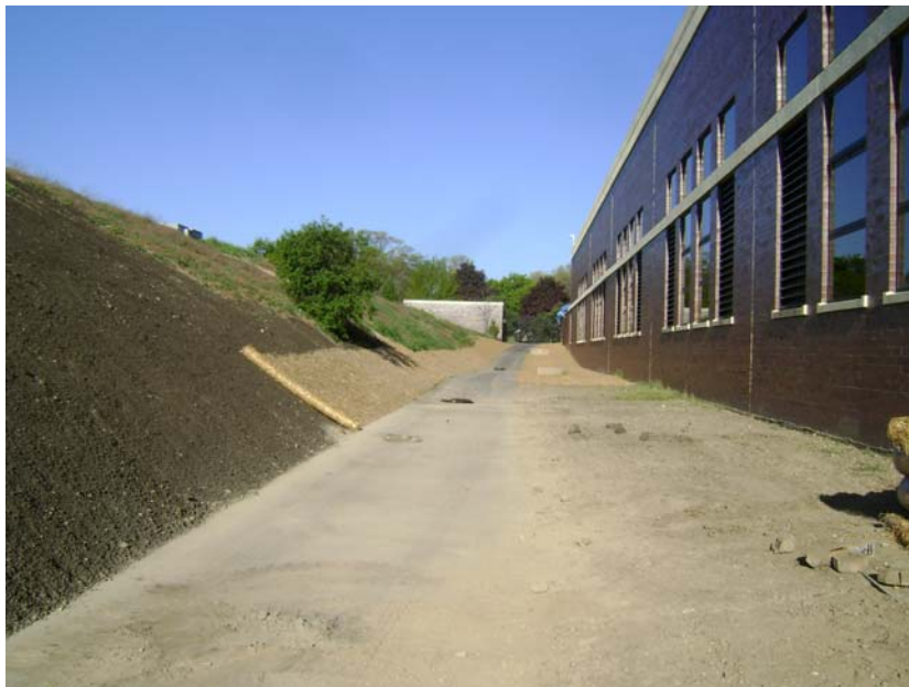
Reservoir Slope Repair
