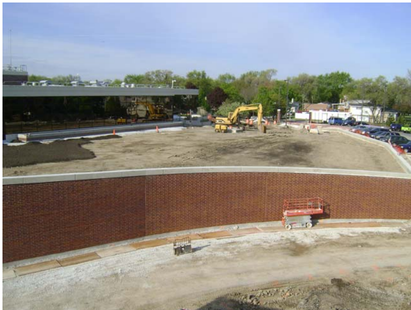
Retaining Wall and Covered Parking Structure Backfill
