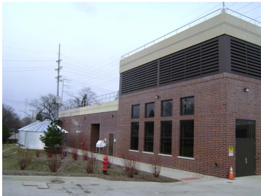
West Face of New Generator Building
