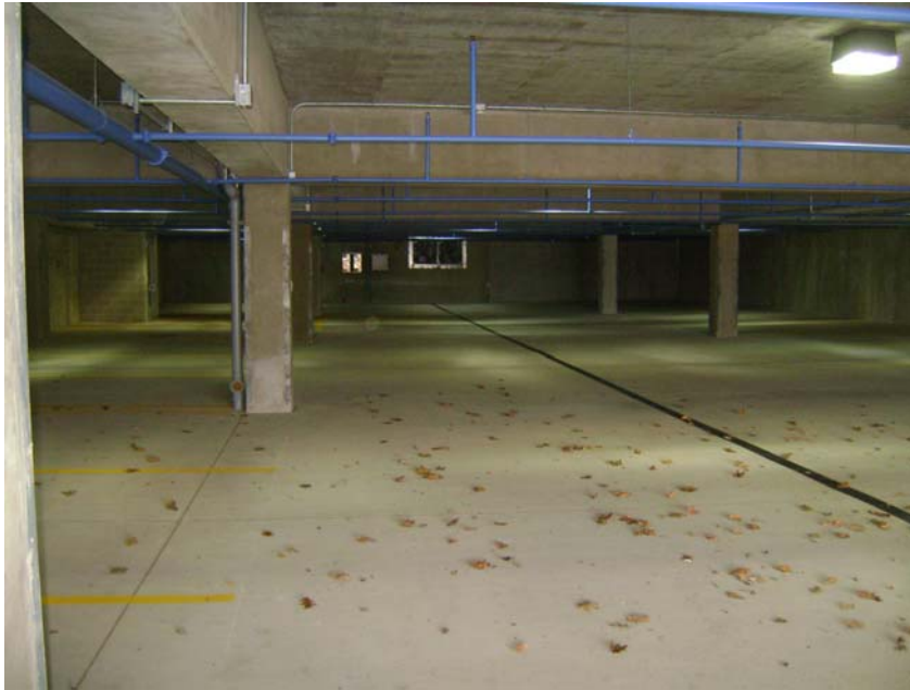
Covered Parking Structure
