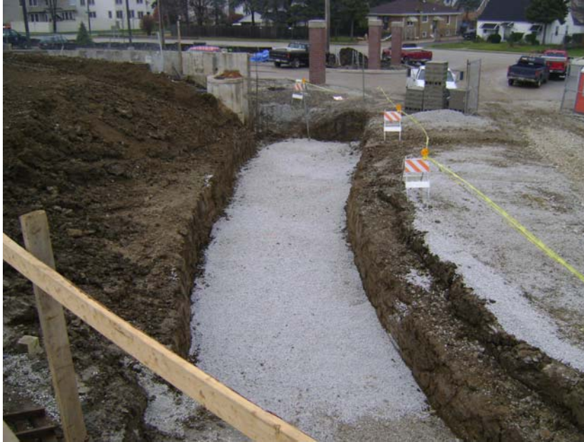
Retaining Wall Footing Excavation
