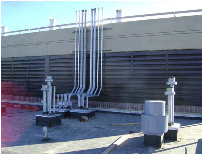
Lube and Fuel Oil Rooftop Vents
