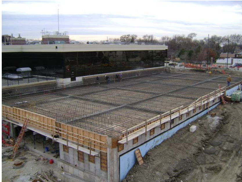
Covered Parking Structure Roof Slab Rebar
