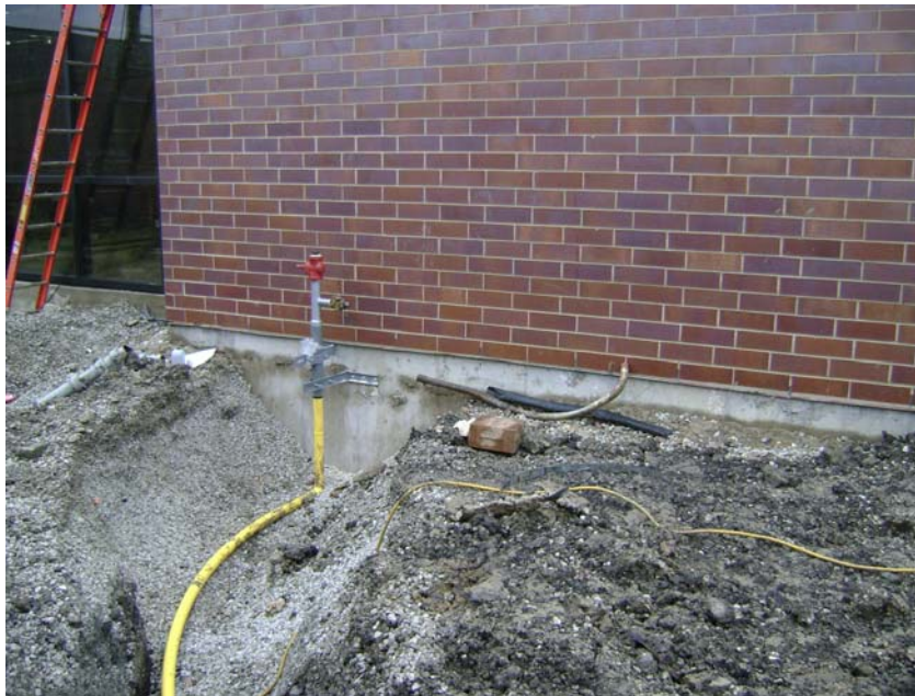
Natural Gas Supply Pipe Installation
