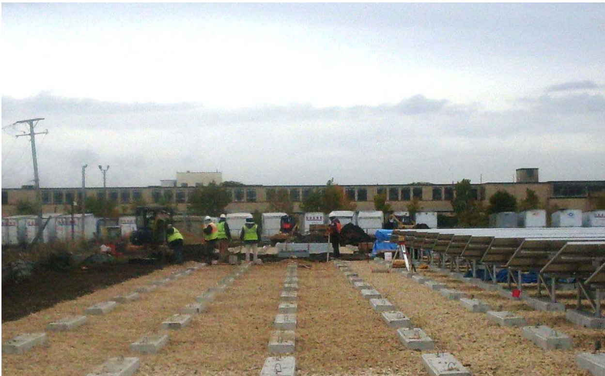
October 14, 2009 Last of the PCP and Stone installation
