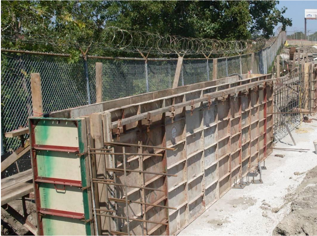
Electrical Building North Foundation Wall Installation
