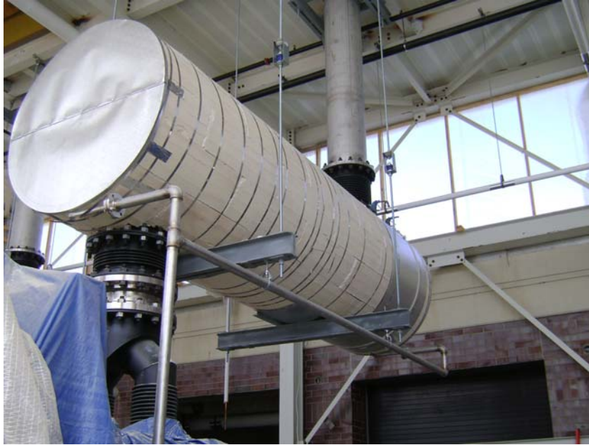
Generator Silencer Insulation Progress
