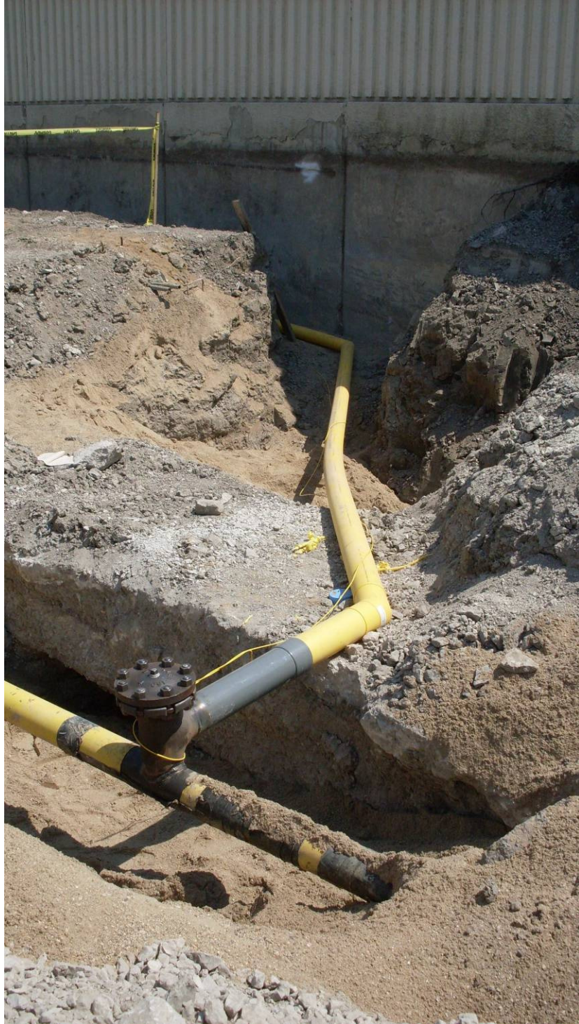
New Gas Main Tie Point Prior to Final Connection
