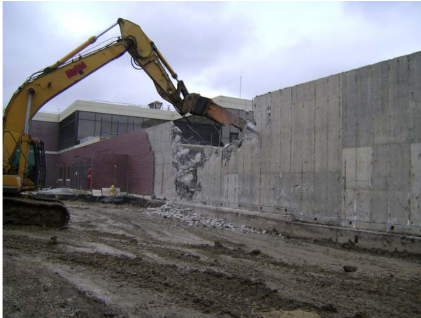
Demolition of Existing Retaining Wall
