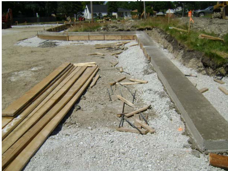
New Parking Lot Curb Construction
