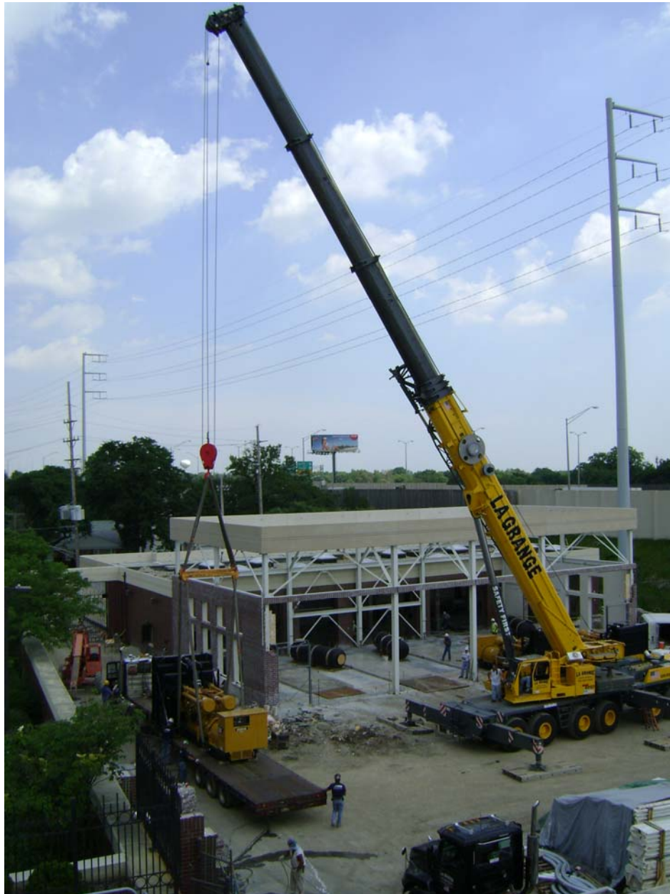
Offloading Engine-Generators Sets
