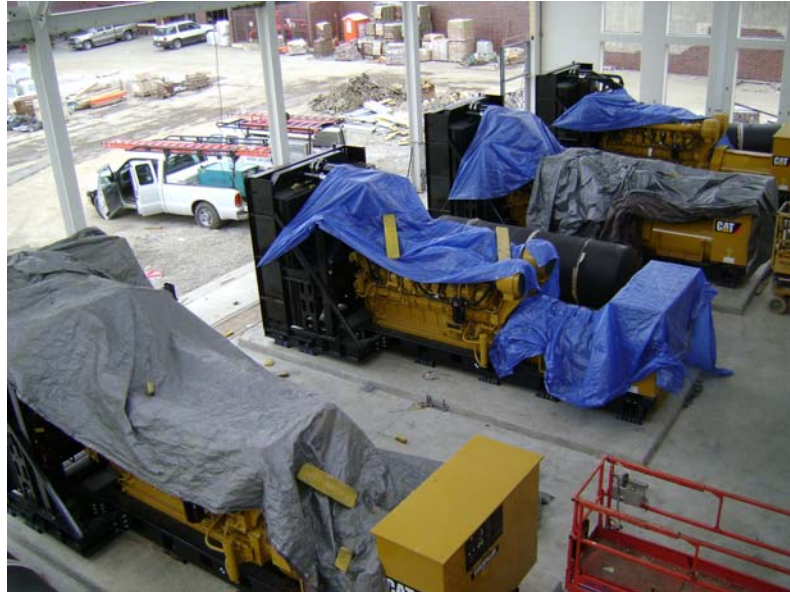
Engine-Generator Sets on Equipment Pads
