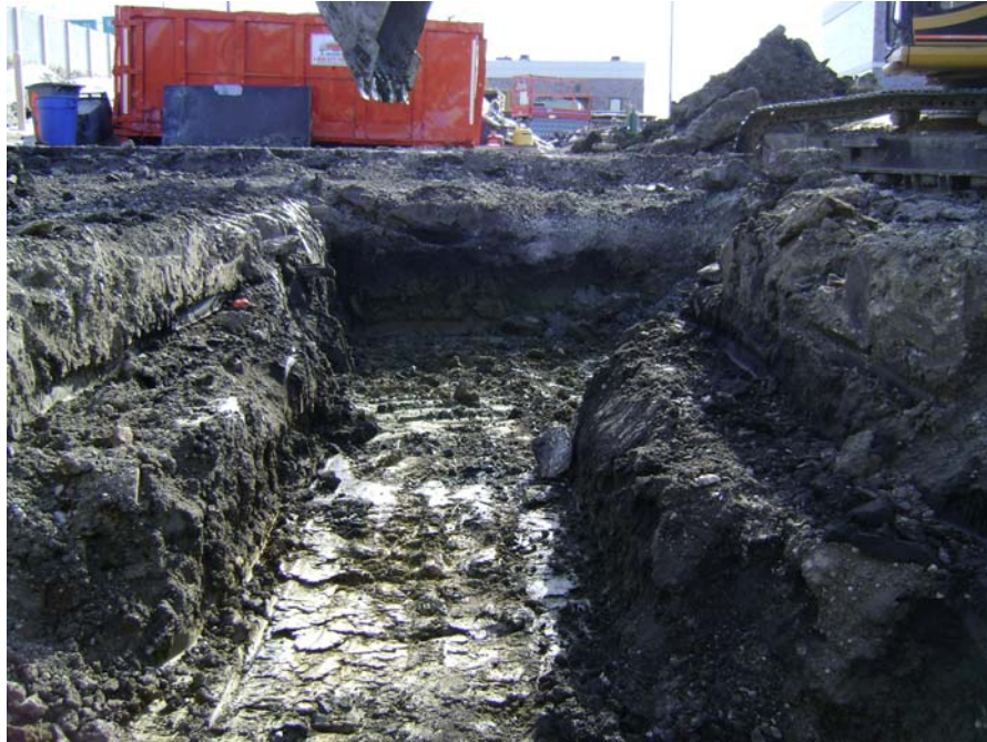
Generator Building Foundation Excavation
