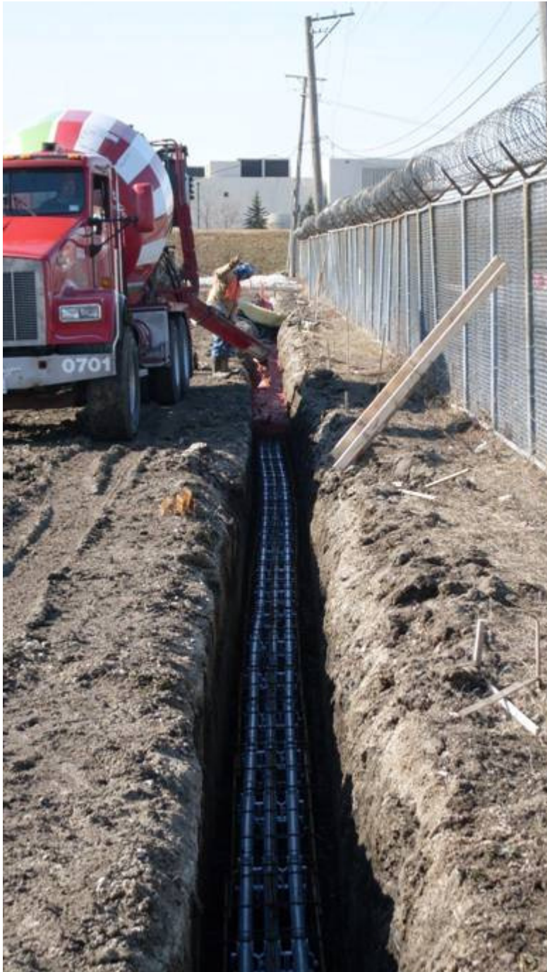
South access road electrical duct bank installation (south of Sec. of State)
