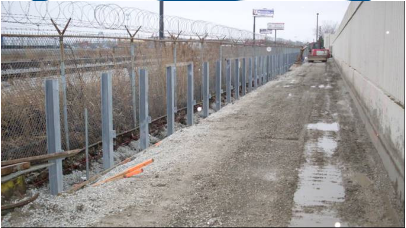
“H”-pile installation for soldier pile retaining wall
