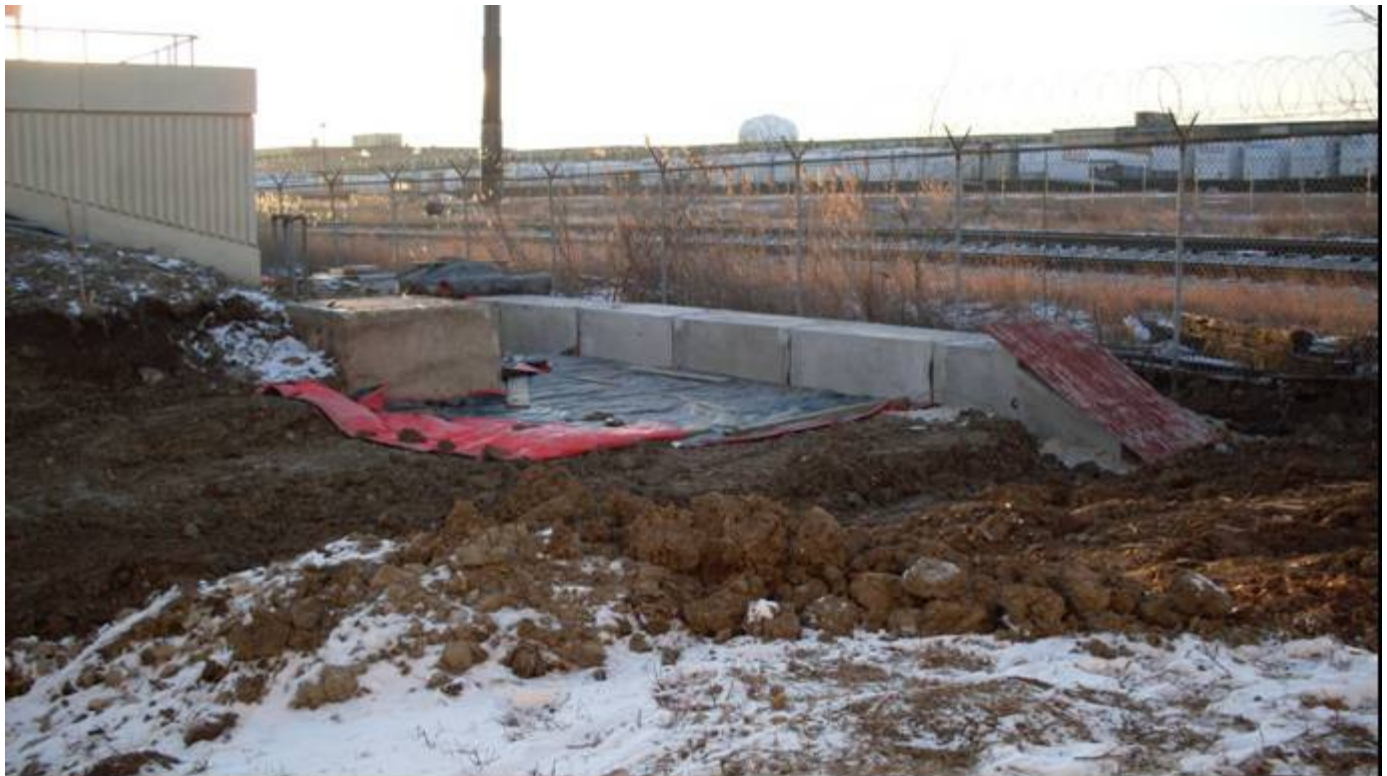
Storm sewer box culvert installed
