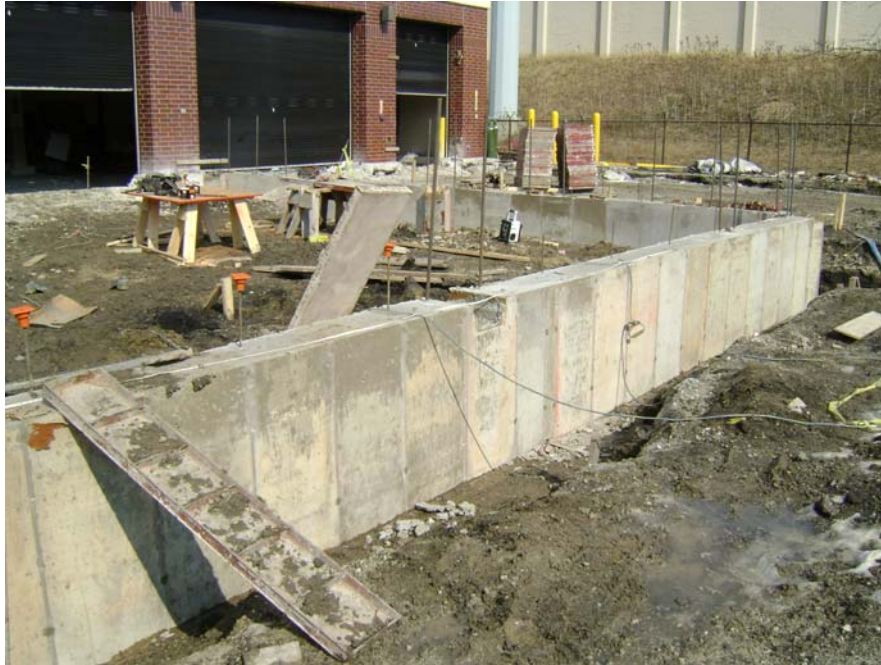
Generator Building Foundation Wall
