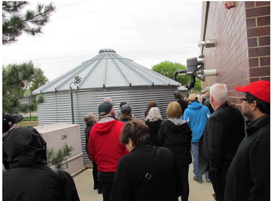
Members viewing the large cisterns that collect water that runs off the green roof of the LEED building
