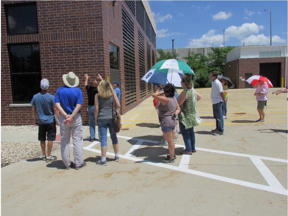
Mike showing the original exterior of the generator building
