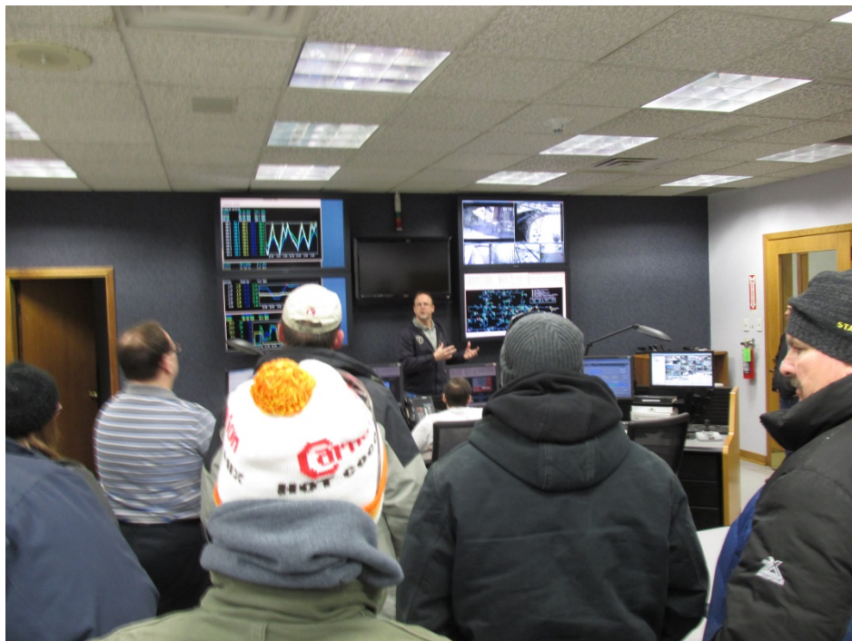
Mike Weed showing DWC's SCADA system in the control room
