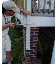
**Step 5.** Put the barrel in place, with the top ring and mosquito screening on top. Re-attach the curved downspout end-piece to the downspout.
