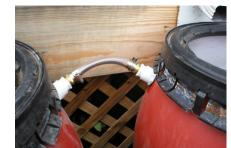
There are many ways to connect one barrel to another. Here, we used some plastic tubing and hose clamps.
