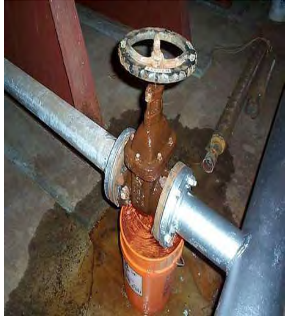
Leaking valve 11
